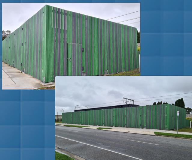
**1** Treadwell's SecurEX® FRP panels are constructed with non-conductivity properties, ensuring safety from potential stray electrical currents.
